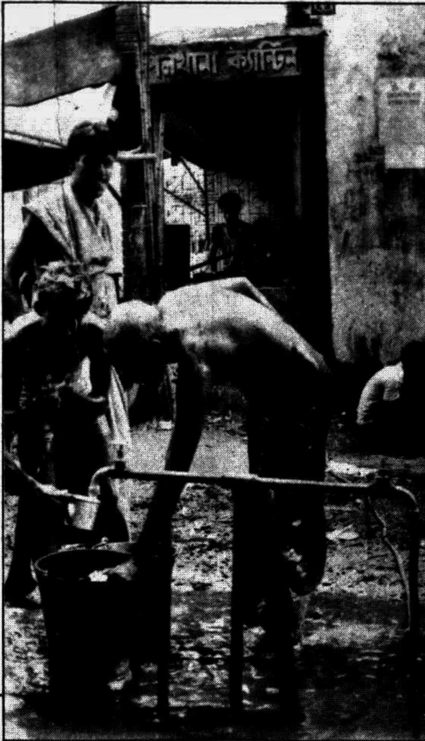
A restaurant near BDR auditorium at Peelkhana drawing water illegally from a public tap through a plastic pipe. — Star photo
