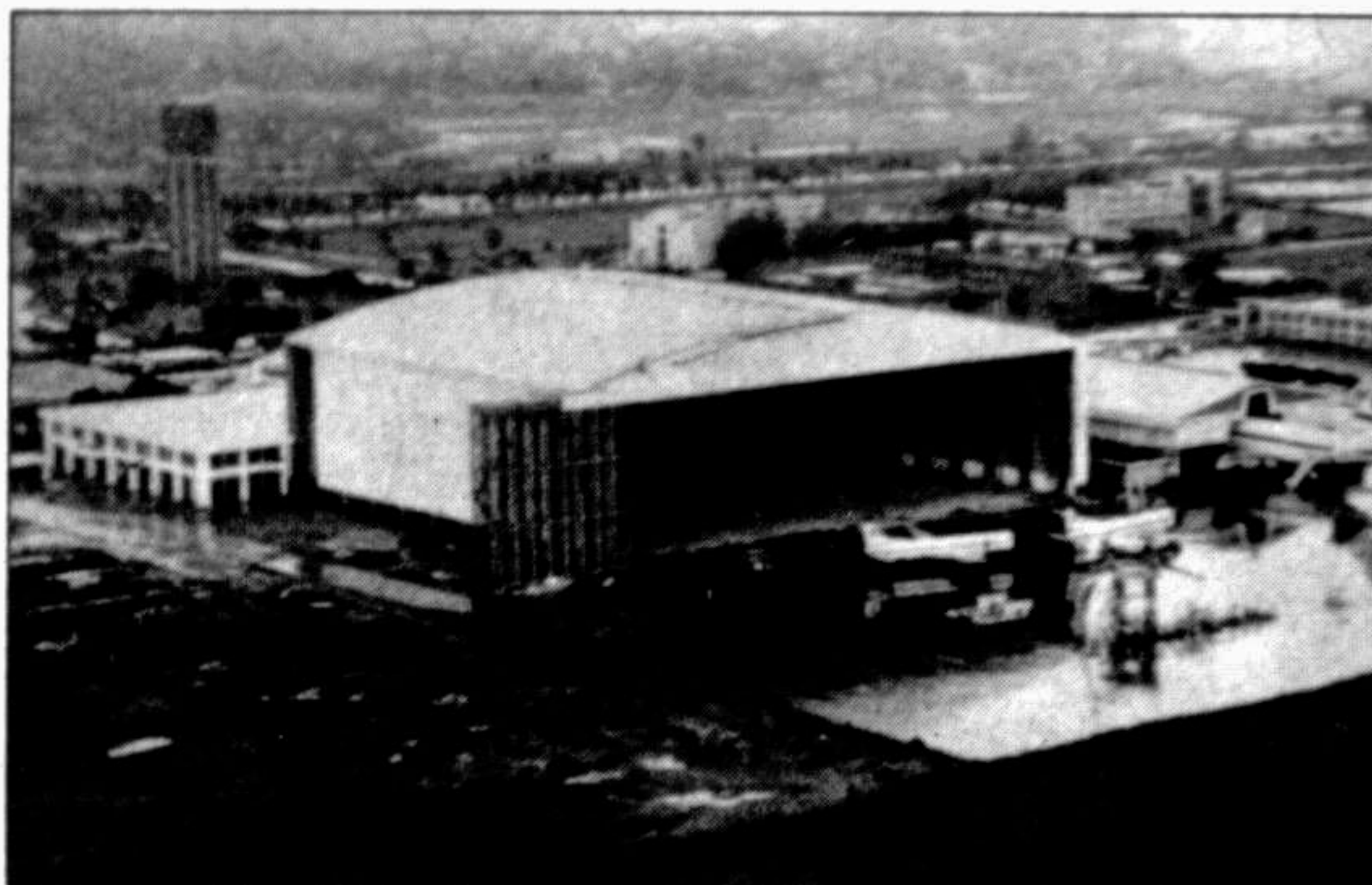
Biman Bangladesh Airlines is implementing its Maintenance and Hangar Complex Project which is nearing completion. The 29,528 million US Dollar Hangar Complex is a full 'turn-key' project which includes finance, design, documentation, procurement, construction, commissioning and training of the local workforce.
