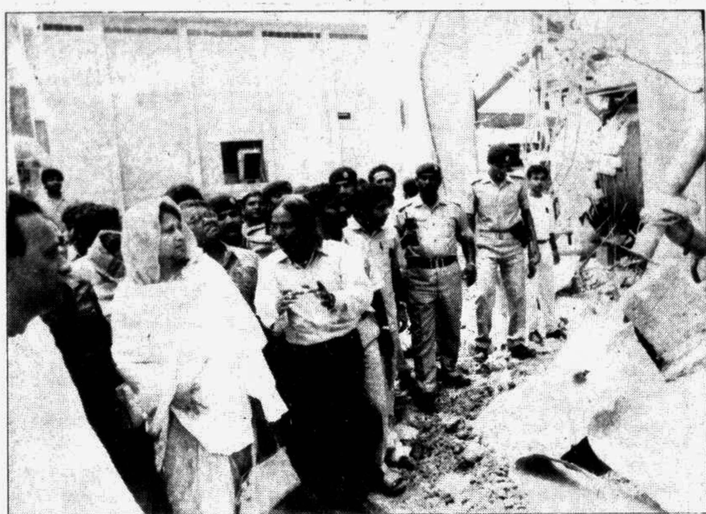
Prime Minister Begum Khaleda Zia visiting the damaged ammonia plant of the Ghorasal Urea Fertiliser Factory on Saturday. —PID photo
