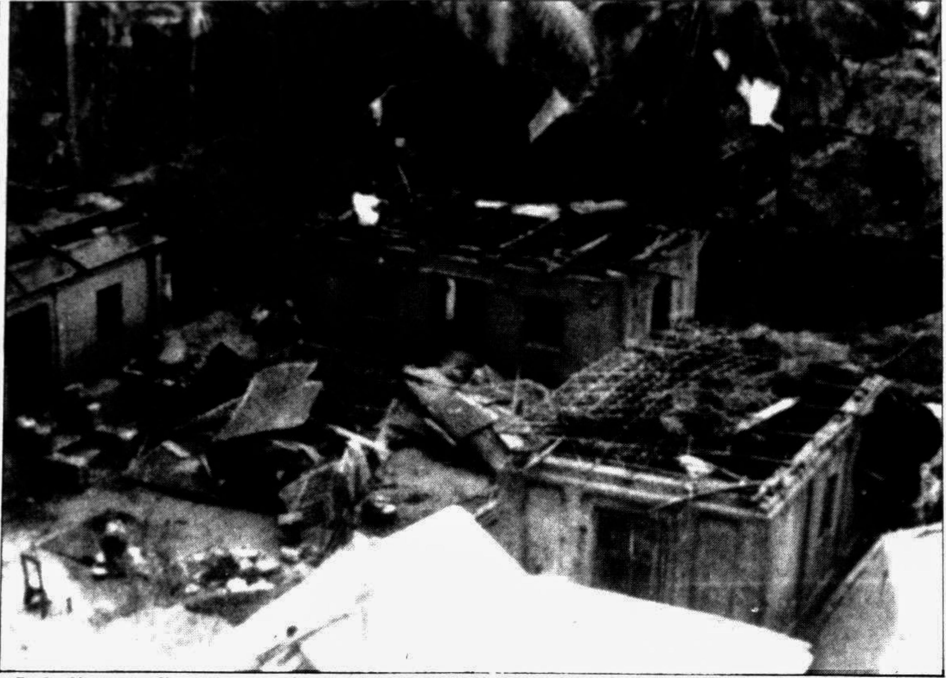
Roofs of houses in Champknagar village of Comilla were blown away in Sunday's tornado. —Star photo
