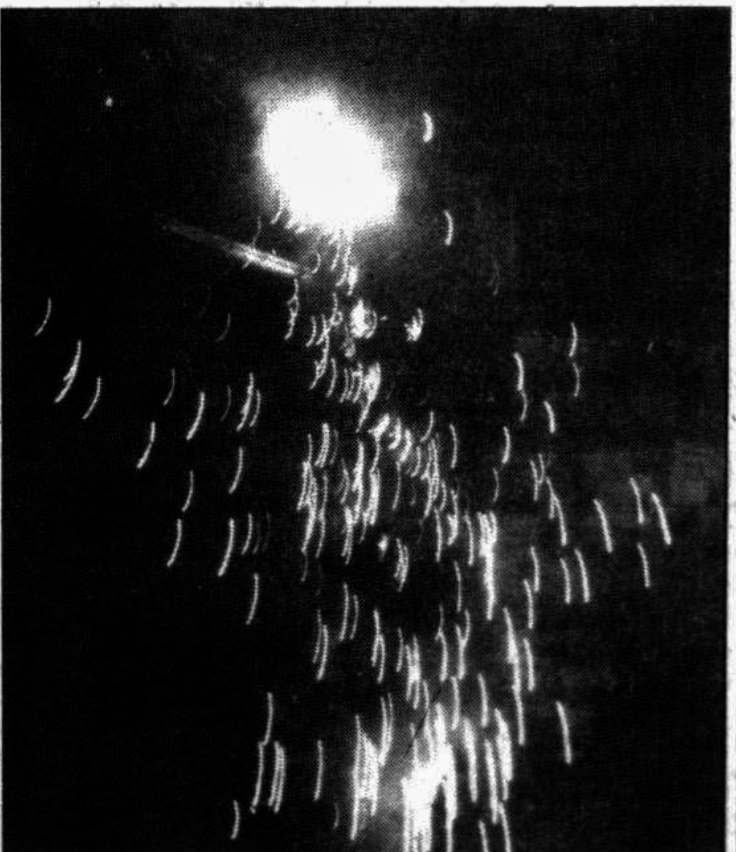
Entire Fakirapool area in city plunged into darkness following electric short circuit on Saturday night. The Fire Brigade personnel, however, came when the damage was done. Huge electric accessories were damaged. Seen in the Star photo is the short circuit.
