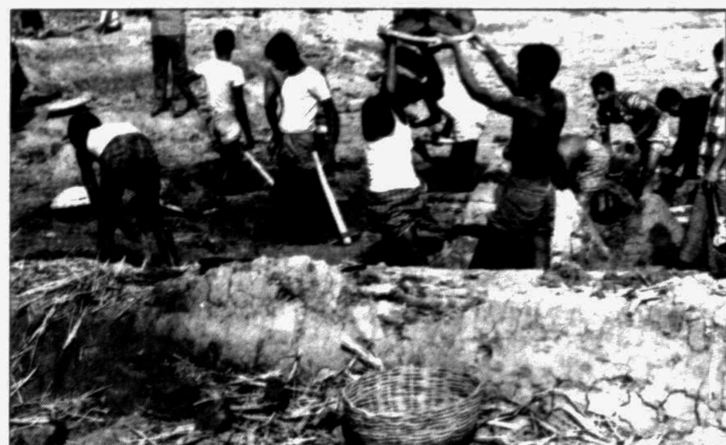
Canal digging in progress in the villages of Bangladesh.
