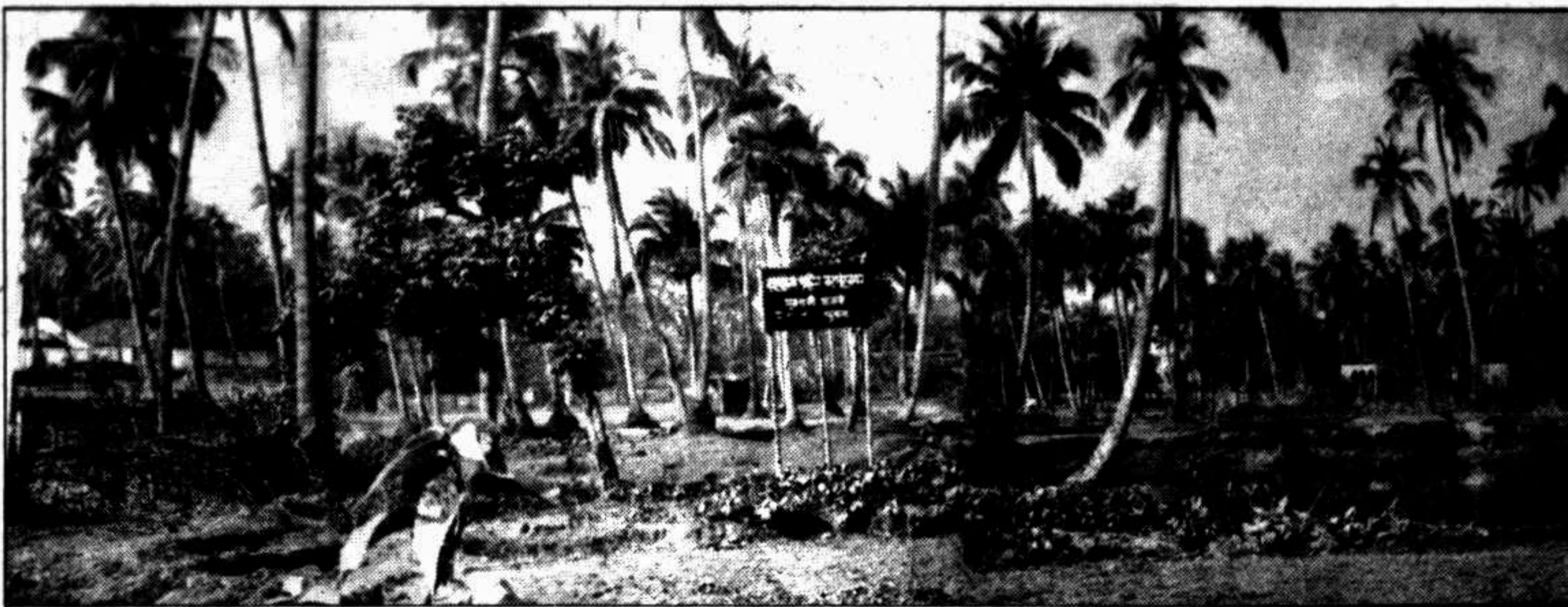
KHULNA: A view of the site selected to construct a motel 23 years ago at a place three miles off the town to develop tourism in the region is lying uncared for. — Star photo
