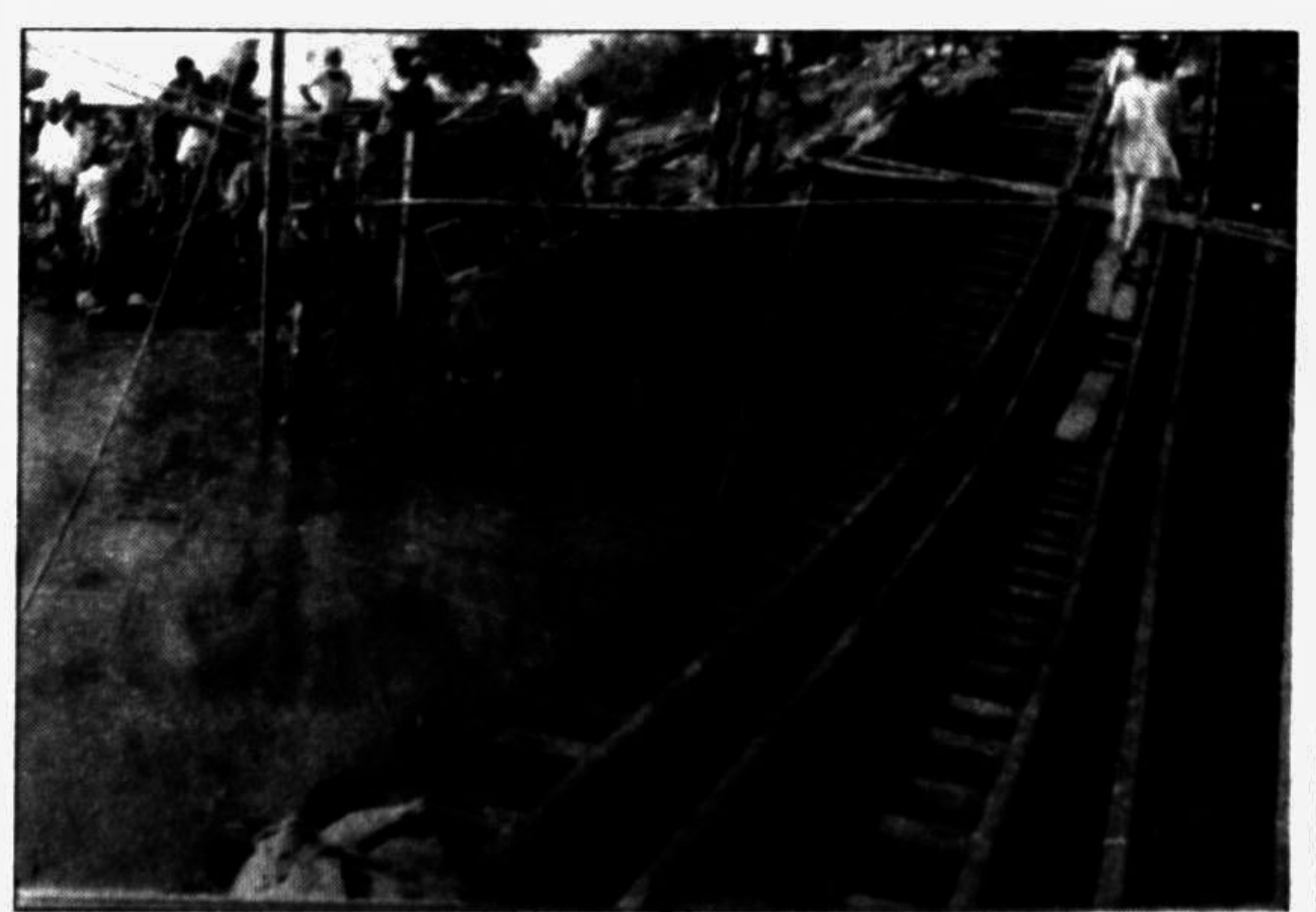
Railway Engineers and workers are engaged in repairing a flood damaged rail-bridge on Teesta-Kurigram section.
