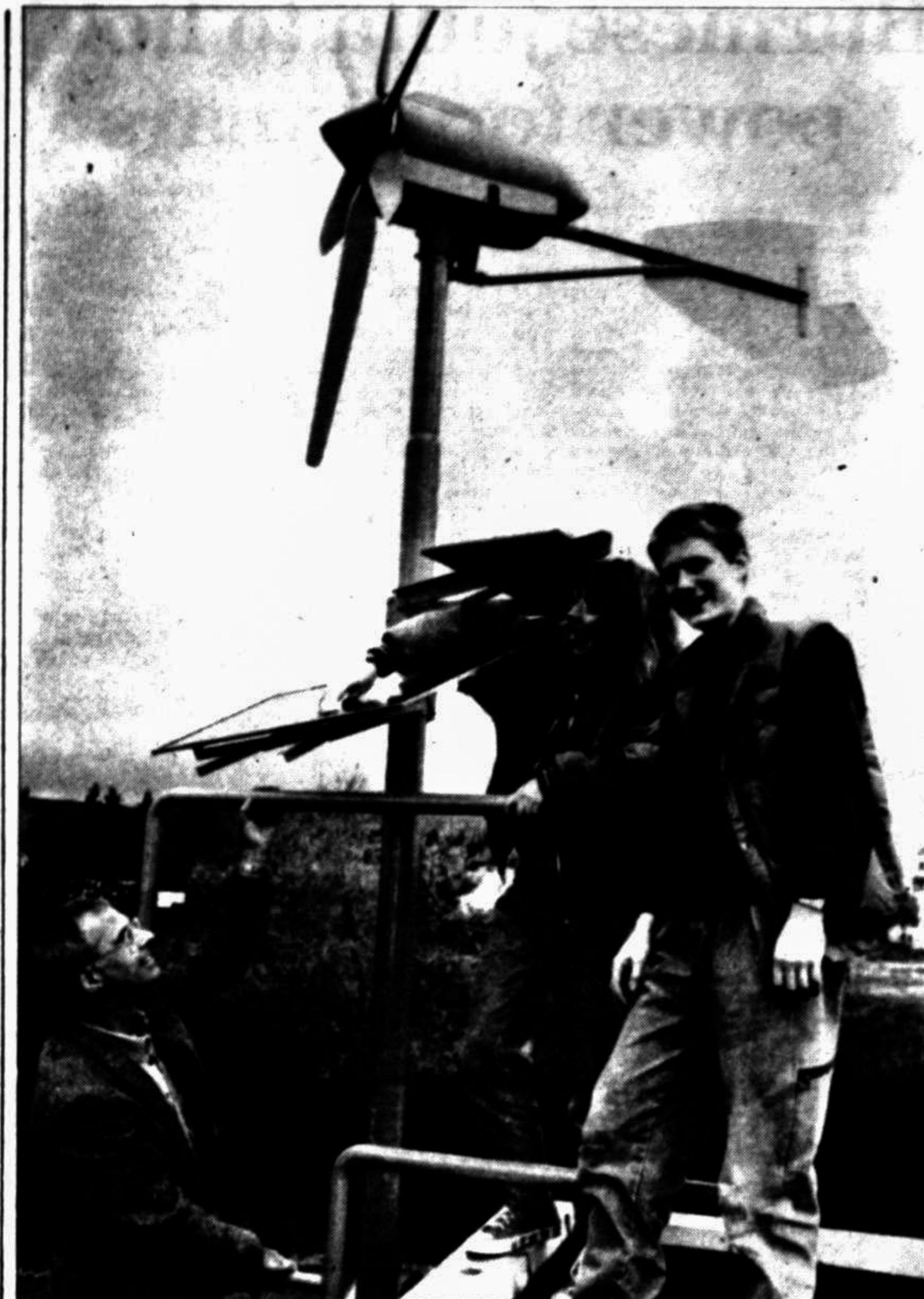
In Kronburg (near Frankfurt/Main), students and teachers built both a wind power and a solar energy facility on the school roof without outside help to supply their science tract with power. —Photo: IN-Press
