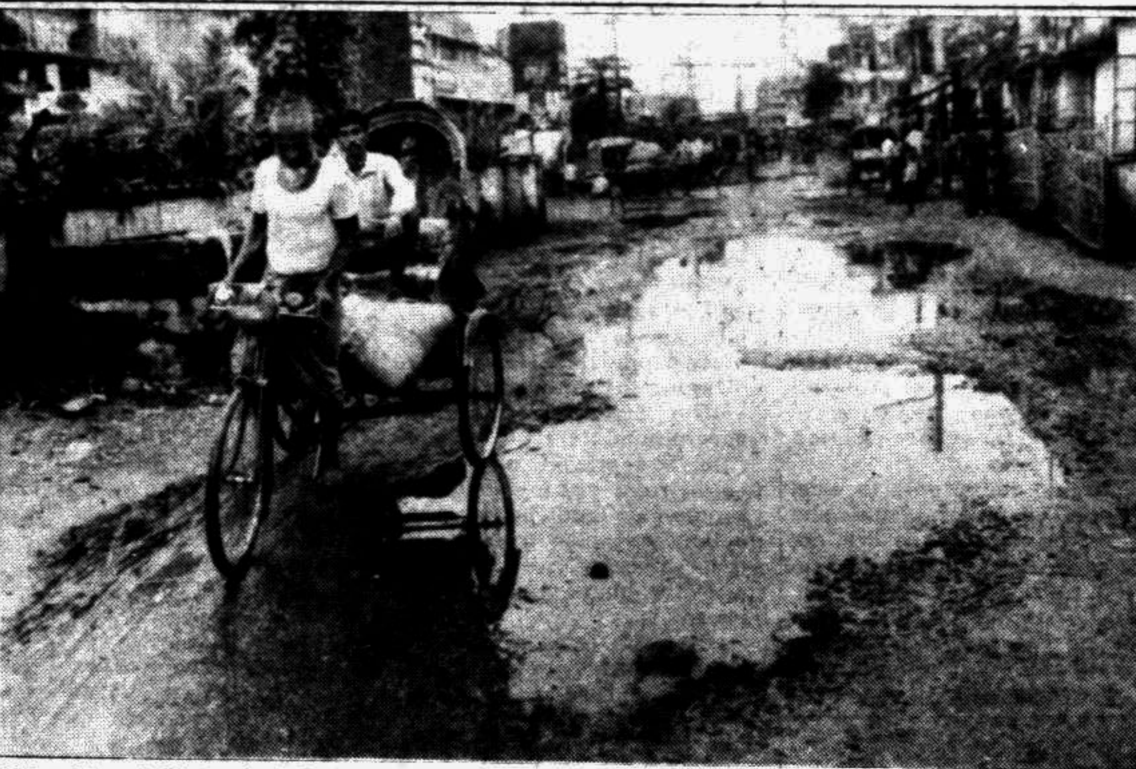
Dilapidated Tajmahal Road in Mohammadpur is causing inconvenience to traffic and pedestrians movement. — Star photo
