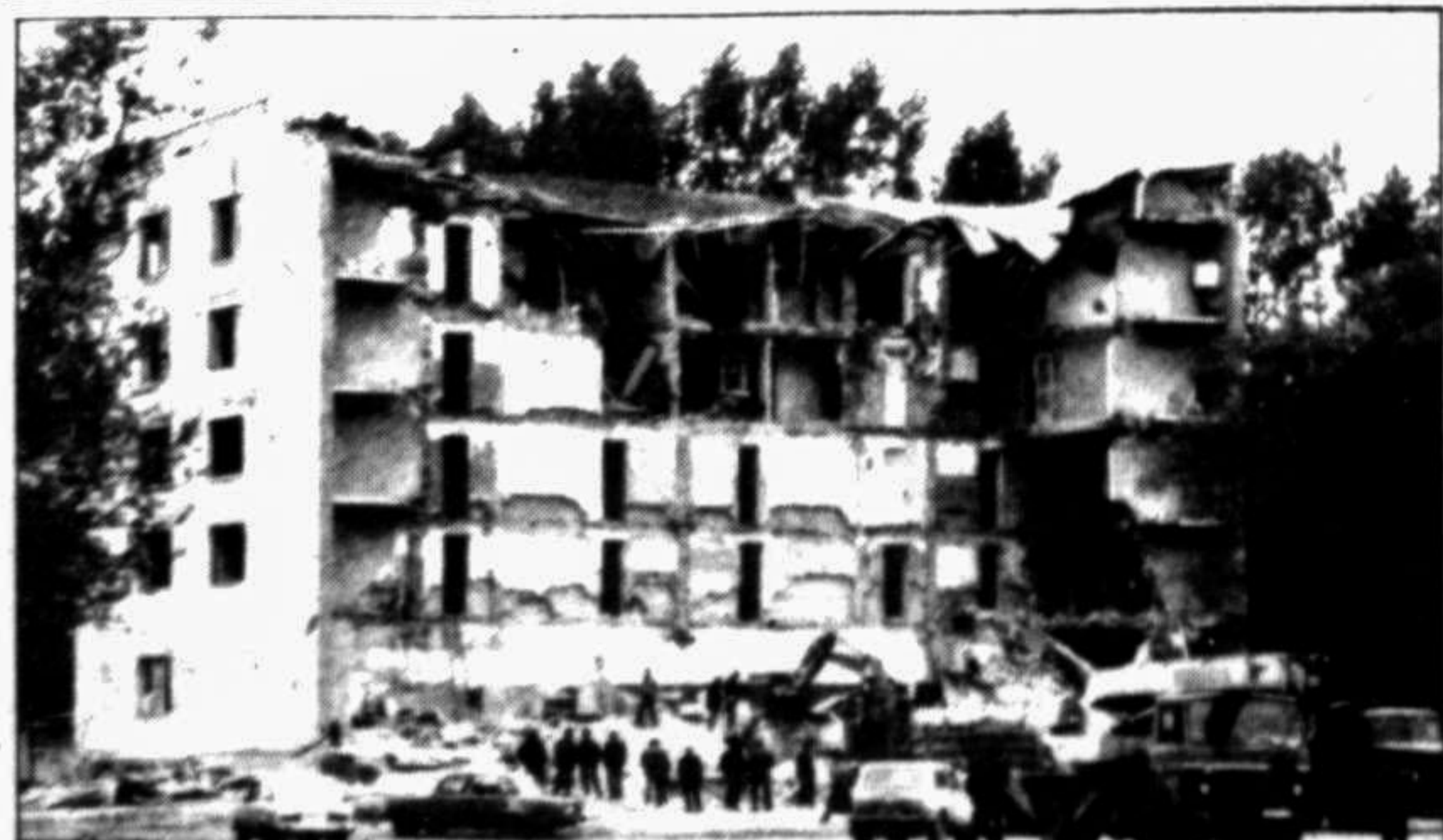
MOSCOW: A dwelling in the town of Taireteli wrecked by the earthquake. — Novosti photo
