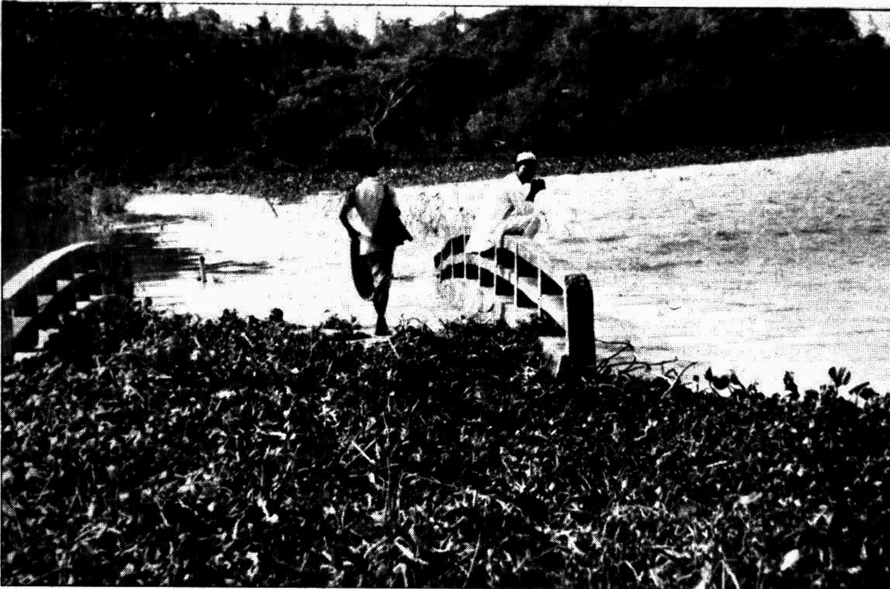
The road between Amura and Kanshiyal unions under Golapganj upazila in Sylhet has been submerged by the recent flood waters. Only this culvert remains a little above water. — Star photo
