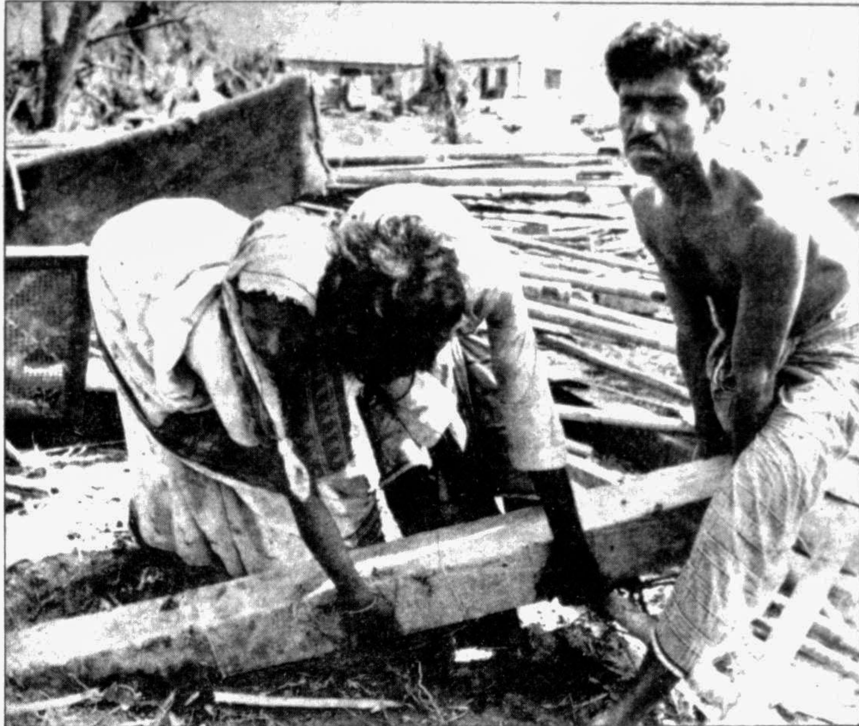
Cyclone survivors with regained will for starting life anew are trying to recover from the debris whatever left to reconstruct their homes. — Star photo
