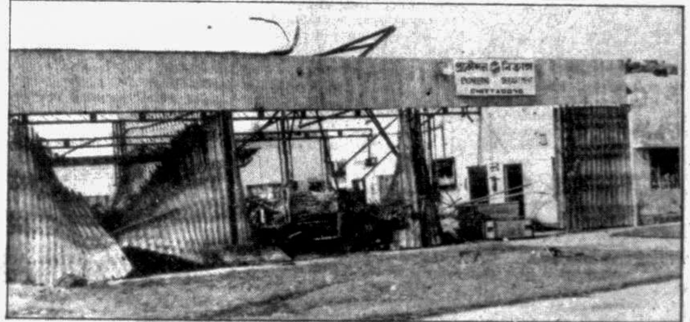
A partial view of Patenga Airport in ruins.
