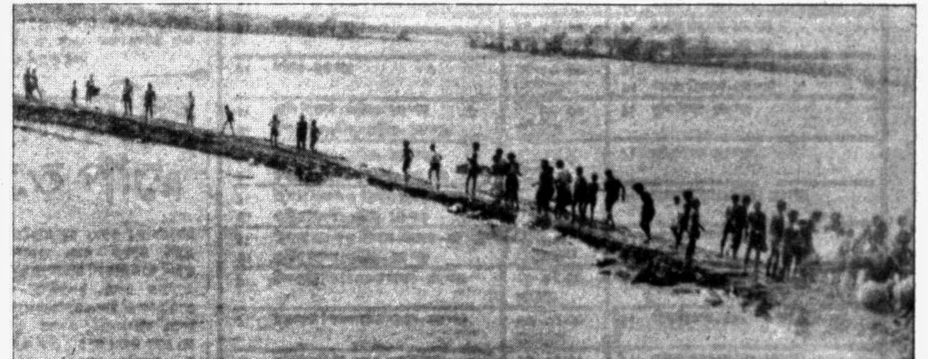
Fortunate survivors of Monday night's catastrophic cyclone in Kutubdia island have nothing but an embankment to take shelter on.
