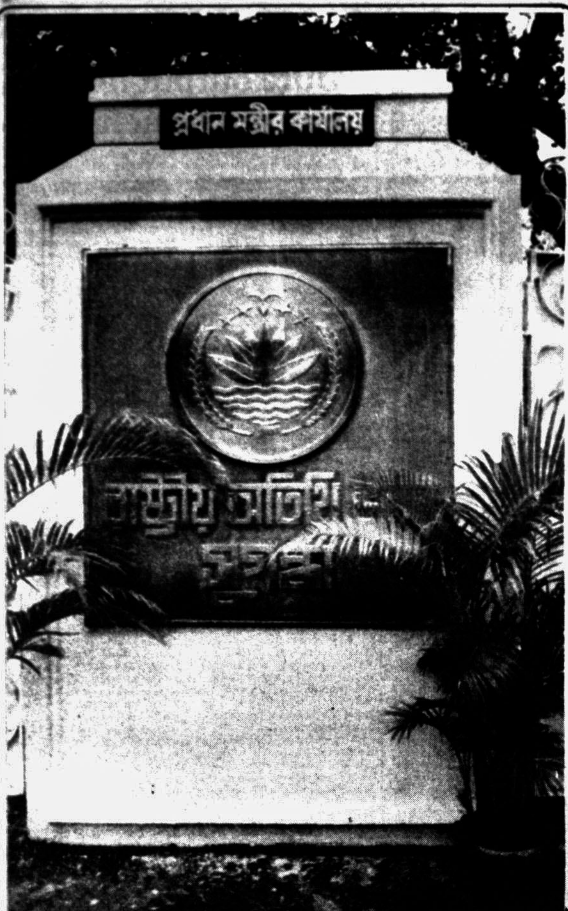
PARADOX PREMIER: Sugandha or the old Ganobhaban is abuzz again with having another Prime Minister but the premier's office-turned-state-guest-house-turned-premier's office building perhaps, now, does double function of hosting state guests and housing the Prime Ministers office. So, at least, say the inscriptions on the main gate. — Star photo
