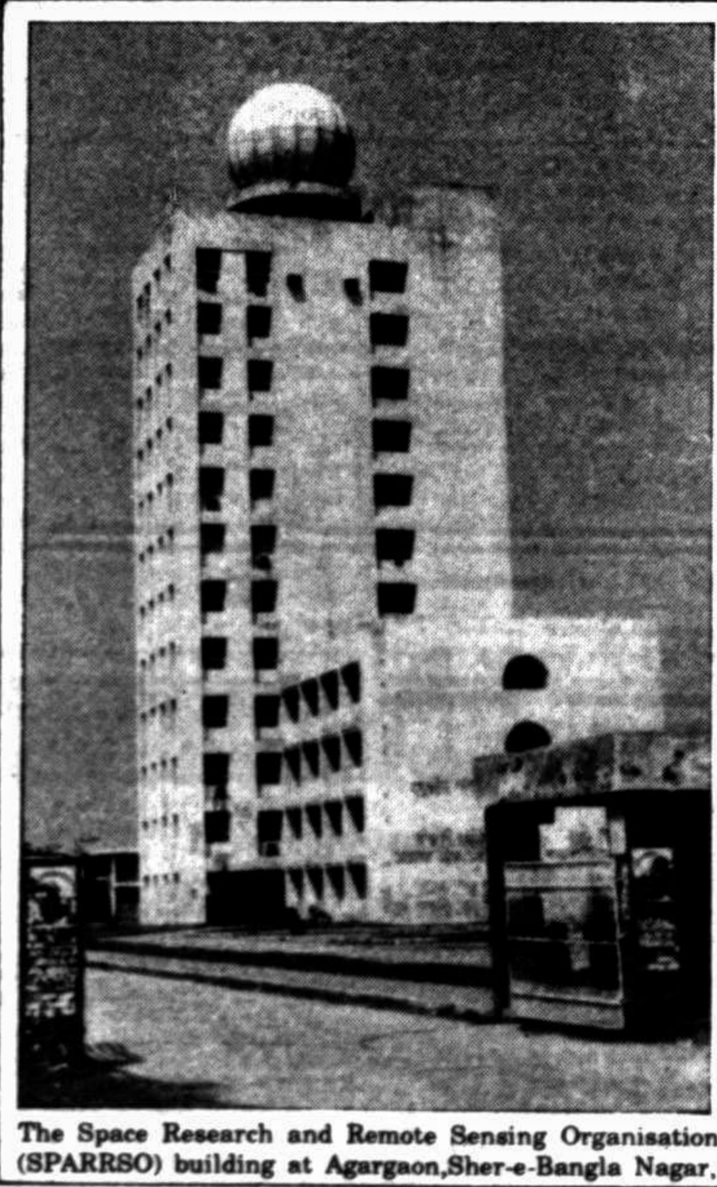
The Space Research and Remote Sensing Organisation (SPARSO) building at Agargaon, Sher-e-Bangla Nagar.
