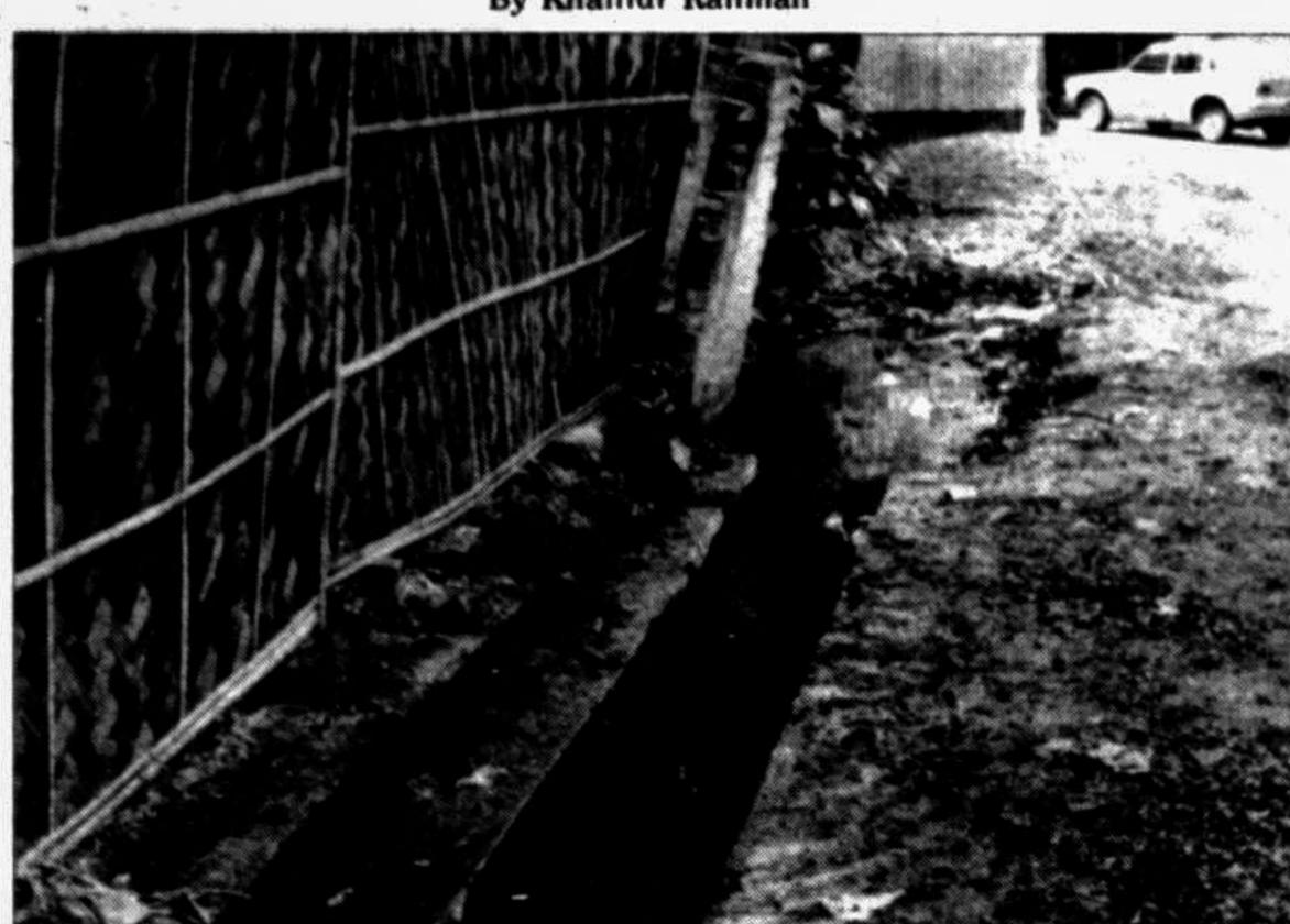
NO WAY OUT: The surface drain, constructed recently by Dhaka City Corporation at Khilgaon, has no outlet. -Star photo
