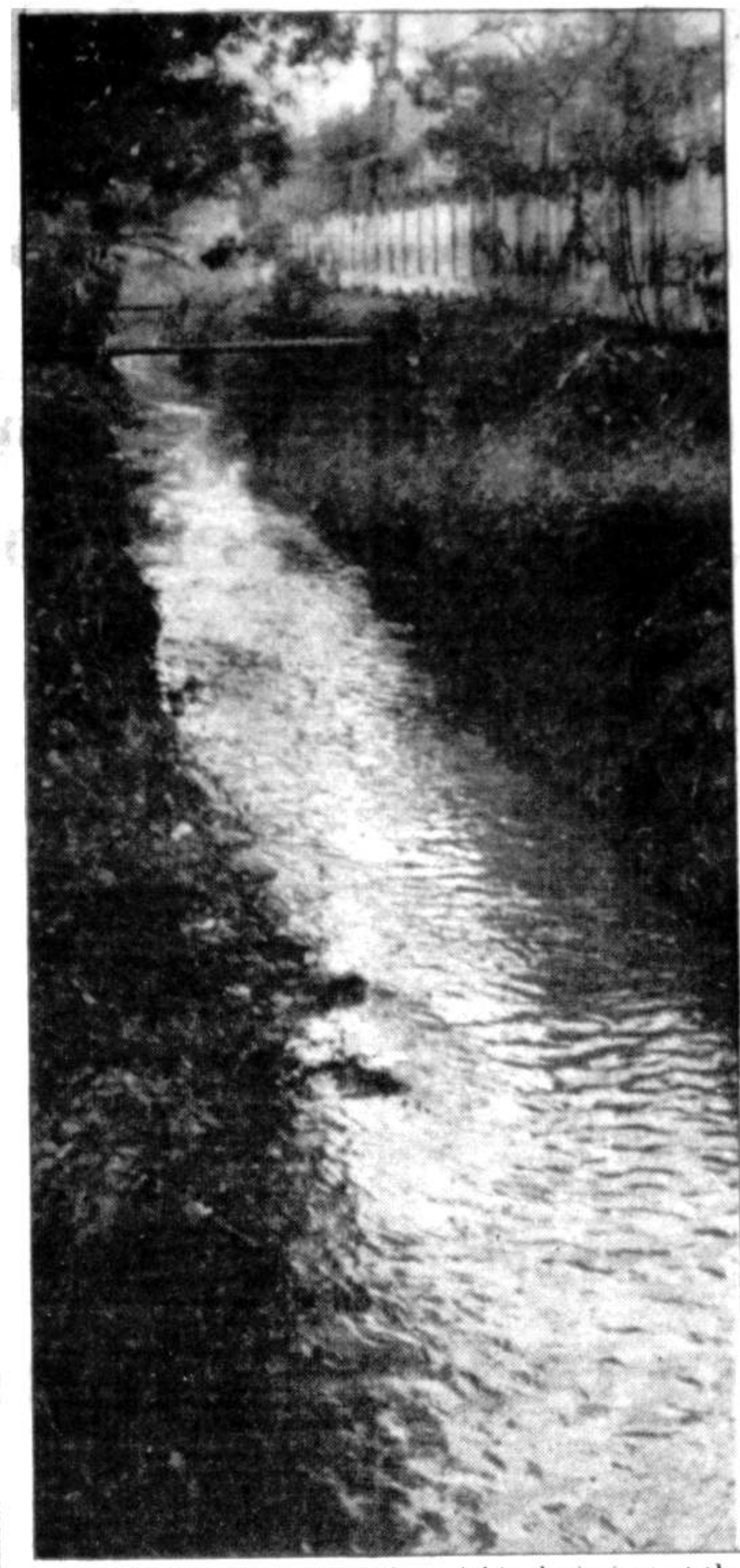
NOT REALLY A CANAL --- A big drain just at the heart of the national capital at Paribagh is without fences to avoid accidents. A rickshaw fell into it on Tuesday, taking its driver and passenger to a dive in soiled water. The drain appears to be nobody's baby ---Star Photo
