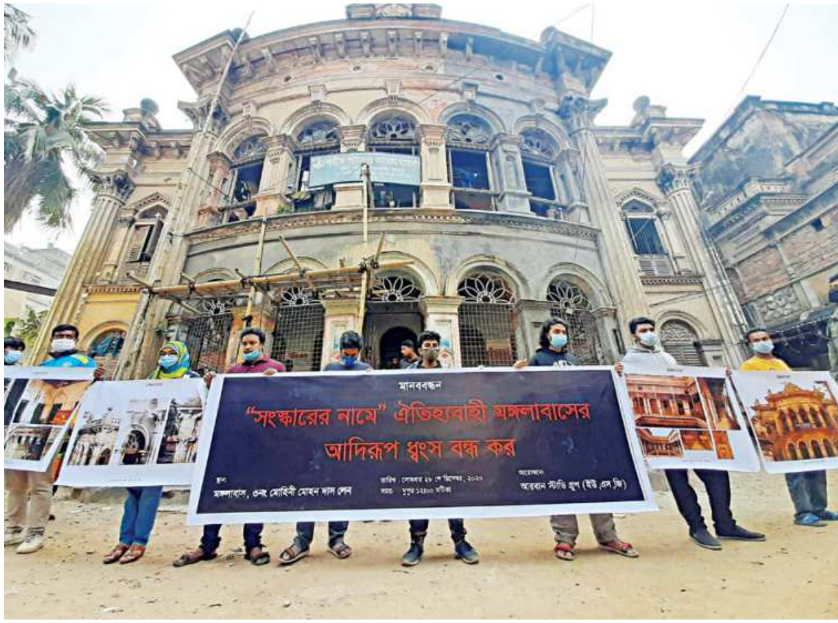
Activists of Urban Study Group gathered in front of Mongolabash in Old Dhaka's Sutrapur yesterday, demanding a stop to the renovation work that puts the structure's heritage at risk.
