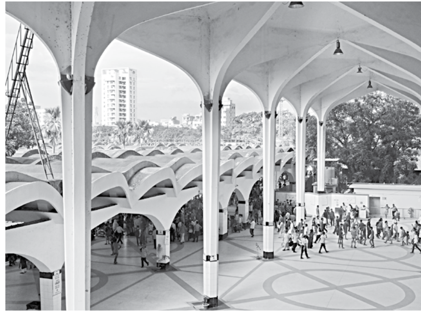
The iconic Kamalapur Railway Station's existing plaza is facing demolition due to a new plan regarding the capital's first metro rail.
