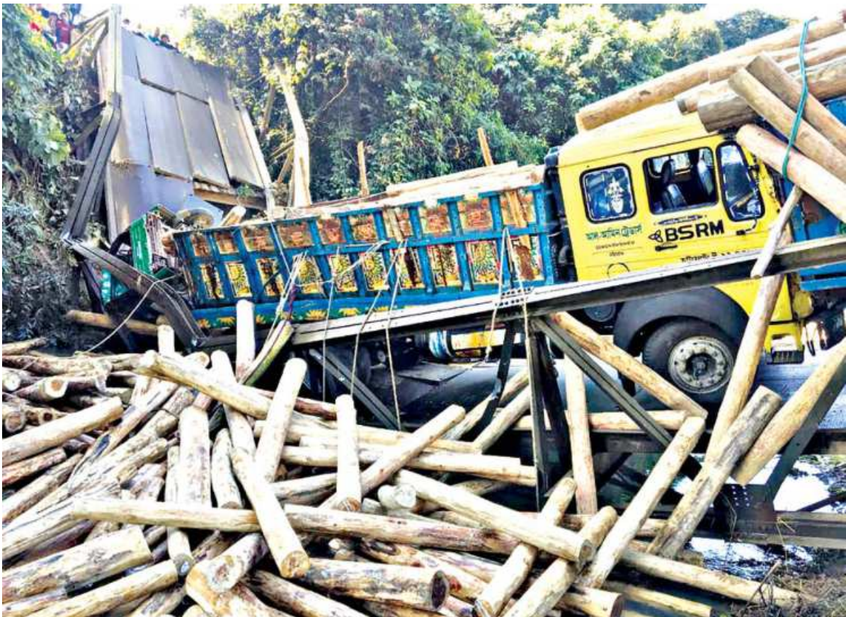
Logs carried by the truck are scattered all over the ditch after a Bailey bridge gave way under the weight of the overloaded truck. A three-wheeler following the truck was the innocent victim. The photo was taken in Khagrachhari’s Dighinala upazila yesterday.
