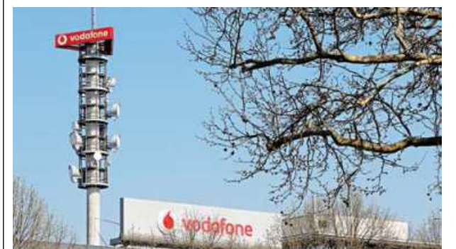
Different types of 4G, 5G and data radio relay antennas for mobile phone networks are pictured on a relay mast operated by Vodafone in Berlin, Germany.
