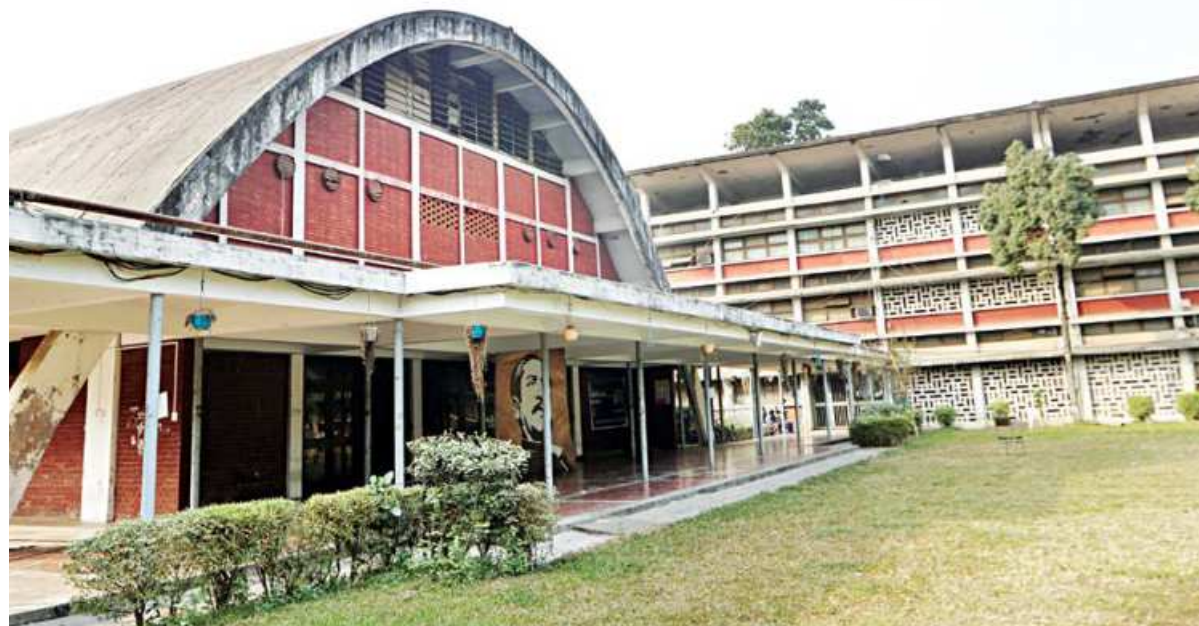
Yesterday's TSC soon to become yesteryear's... This all-too-familiar sight of the red and white dome is set to disappear as the government begins implementing its plan to replace the old TSC structure with a multistoried building.
