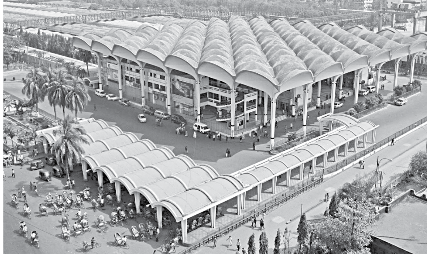
Kamalapur Railway Station.
