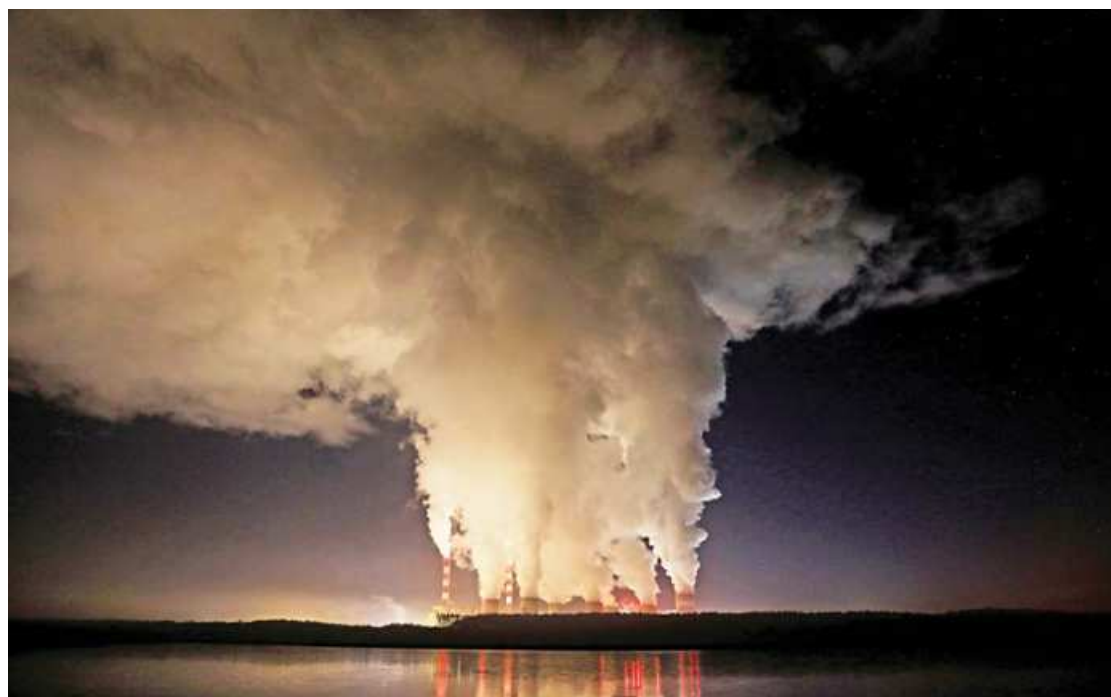
Smoke and steam billow from Belchatow Power Station, Europe's largest coal-fired power plant at night near Belchatow, Poland. Picture taken on December 5, 2018.
