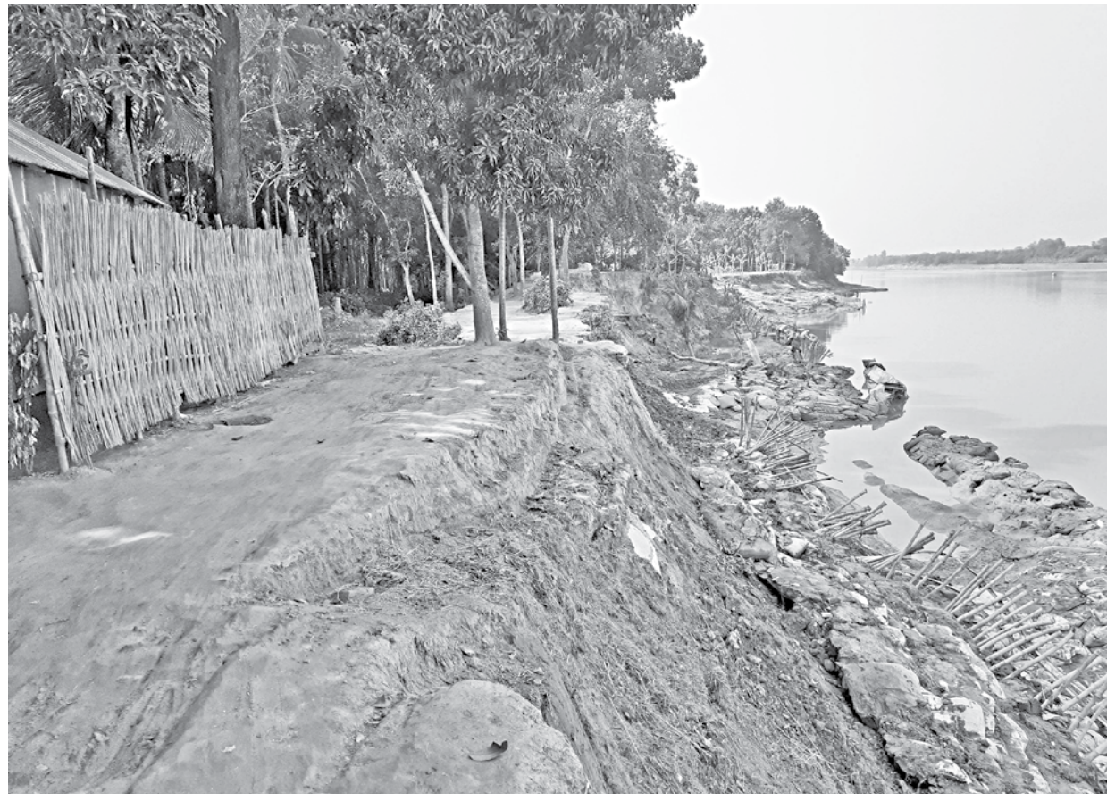
A part of the road, near Bir Shreshtha Shaheed Lance Nayek Munshi Abdur Rouf Library and Memorial Museum in Faridpur's Madhukhali upazila, which was washed away by the Madhumoti river.
