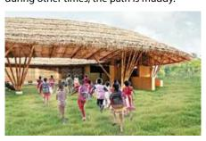
Keeping the landscape in mind, Sonadia School is designed over a raised platform that prevents it from flooding. A channel is connected to the eastern part of the courtyard, through which boats can easily move inside the school.
