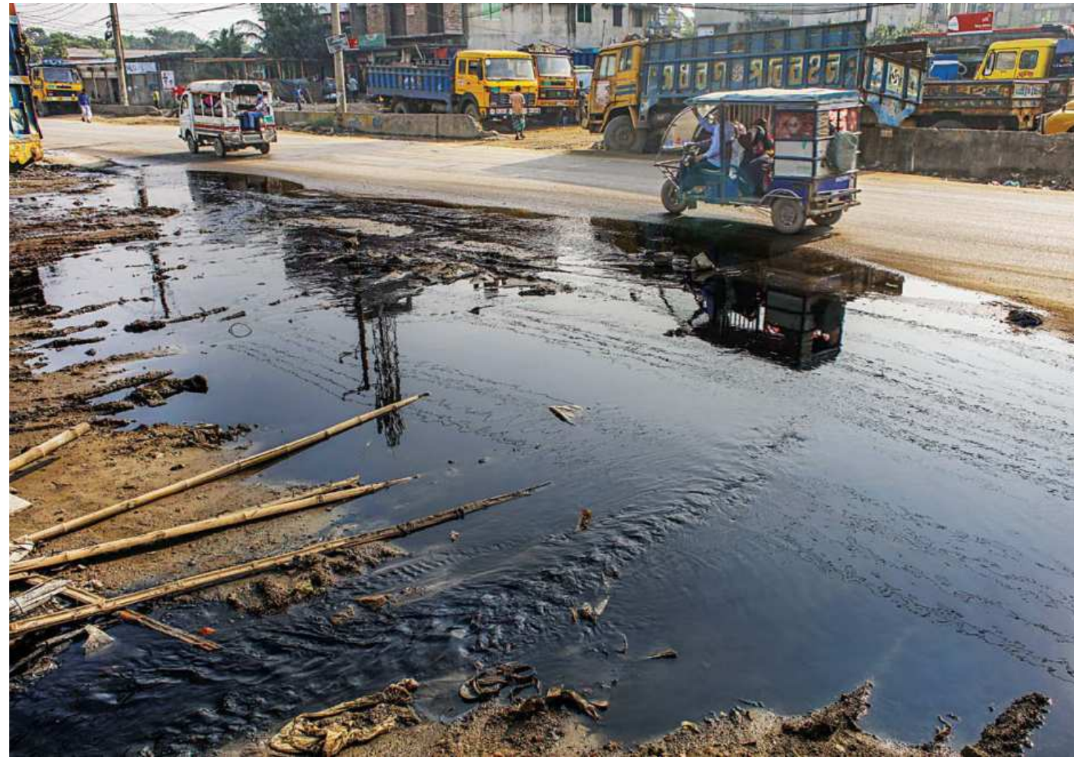
Dirty water from a canal in a WASA-owned water refinery area overflowing onto the Dhaka-Narayanganj road. This has been going on regularly there for the past two months. The photo was taken recently.
