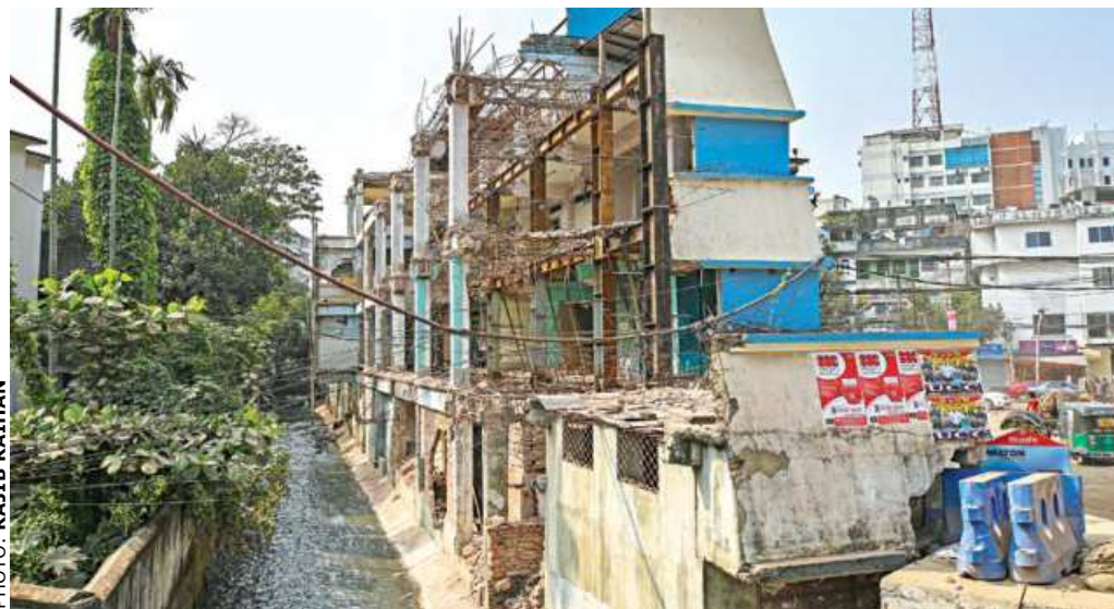
An academic building of Premier University, which was built obstructing a canal in port city's Prabartak mor area, is being demolished to free up the canal. The photo was taken on Thursday.
