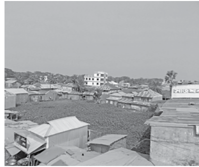
Many illegal structures have been built after filling up a major portion of one of the three government ponds at Mohipur Bazar in Patuakhali's Kalapara upazila.
