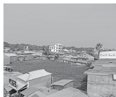
Many illegal structures have been built after filling up a major portion of one of the three government ponds at Mohipur Bazar in Patuakhali's Kalapara upazila.
