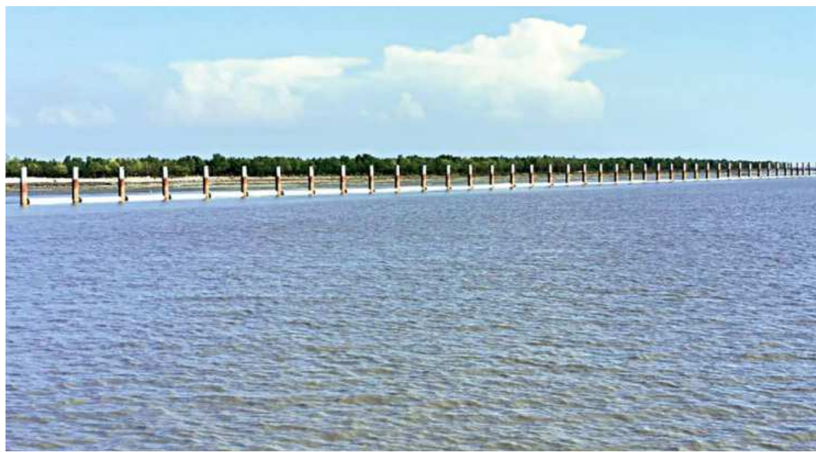
A line of pillars on the embankment of the Bay of Bengal is seen at Bhashanchar island in Nokhali's Hatiya upazila. The four-layer embankment has been built after analysing the data of the last 176 years to protect the inhabitants of the island. The government plans to relocate 100,000 forcibly displaced Rohingyas to this island from the mainland camps of Cox's Bazar. The photo was taken recently.
