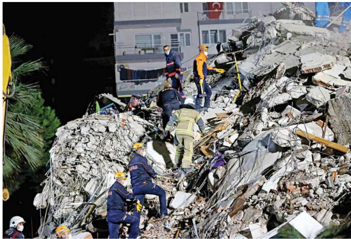
Rescue operations take place on a site yesterday after an earthquake struck near the the coastal province of Izmir, Turkey Killing at least 27 people. At least 20 buildings in Izmir were destroyed, authorities said, and the rescue work was taking place as hundreds of aftershocks hit the area.
