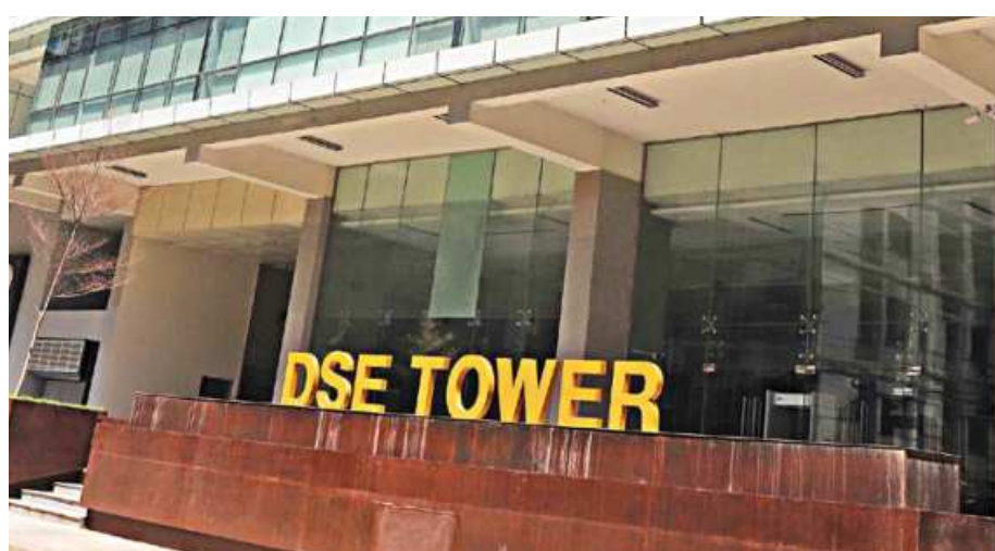
The new headquarters of the country's premier bourse Dhaka Stock Exchange at Nikunja in the capital.
