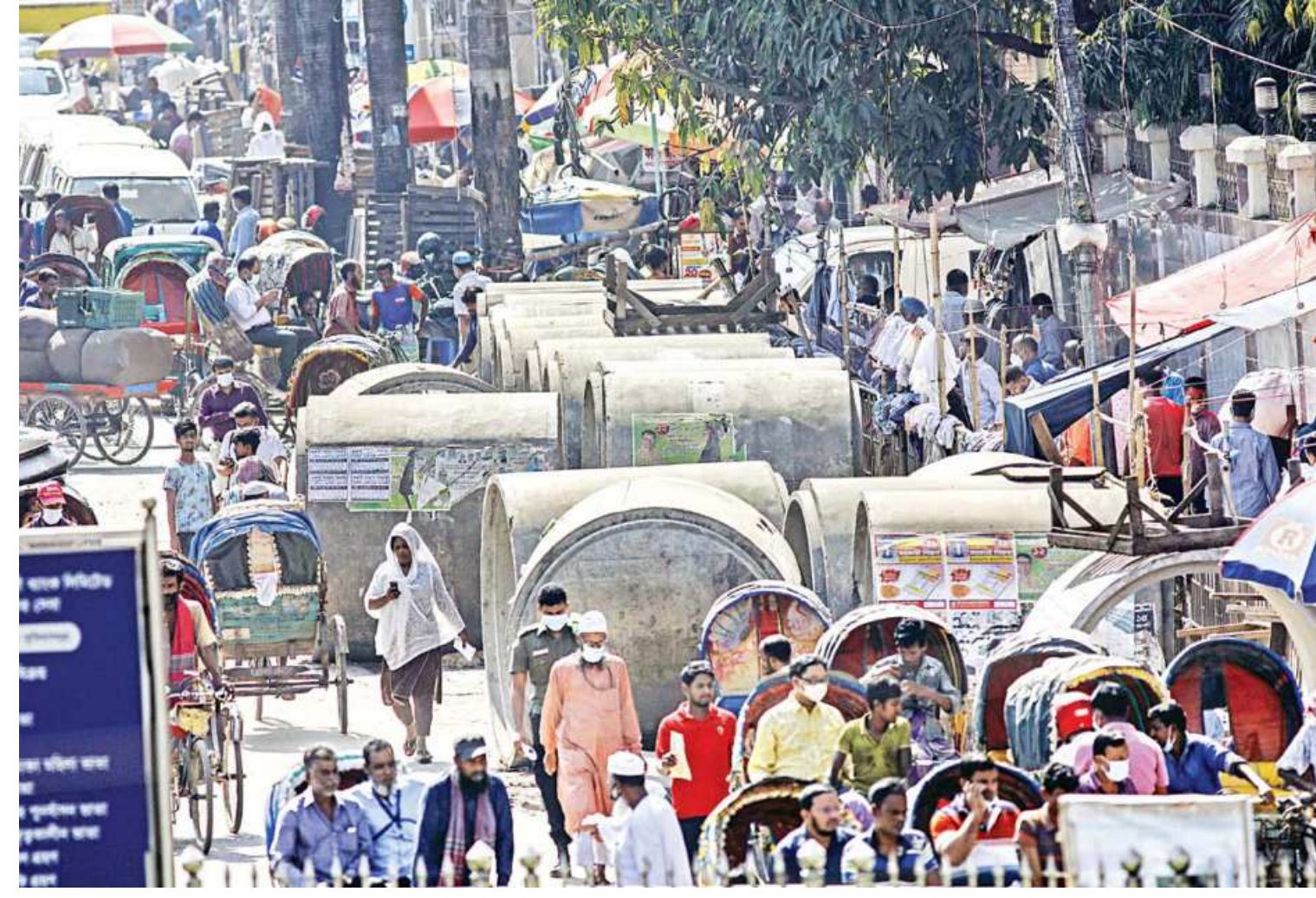
Large concrete pipes of storm-water drain lie right on the street near Bangladesh Bank headquarters in the capital’s Motijheel, obstructing movement of vehicles and pedestrians. Locals said city corporation authorities kept the pipes there for the last eight months. The photo was taken yesterday.
