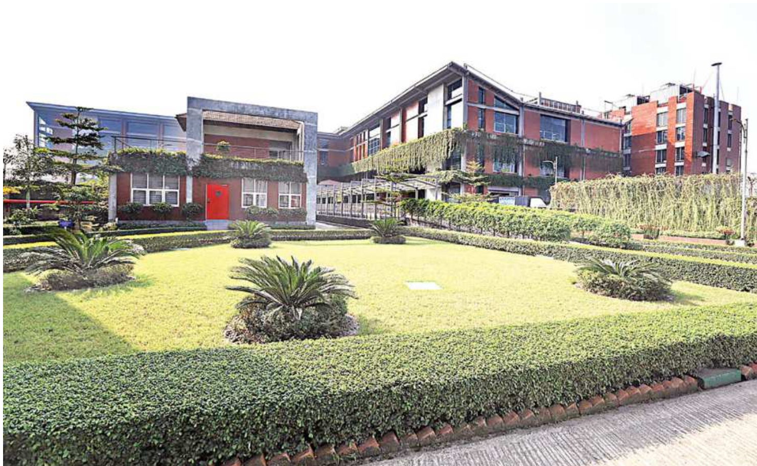
A state-of-the-art green garment factory in Gazipur. Entrepreneurs have to spend 30 per cent more for constructing these factories than the conventional ones.
