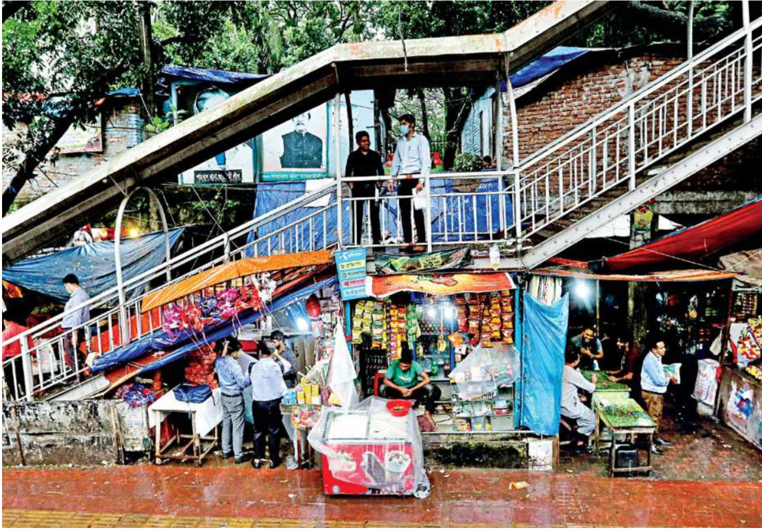
Shops have flourished under the stairs of this footbridge on both sides of the road at the capital's Shahbagh, illegally encroaching all available spaces, some even spilling over to the footpath. Vendors are comfortably running their businesses like this for ages, as authorities seem to turn a blind eye to this open violation. This photo was taken on Saturday.
