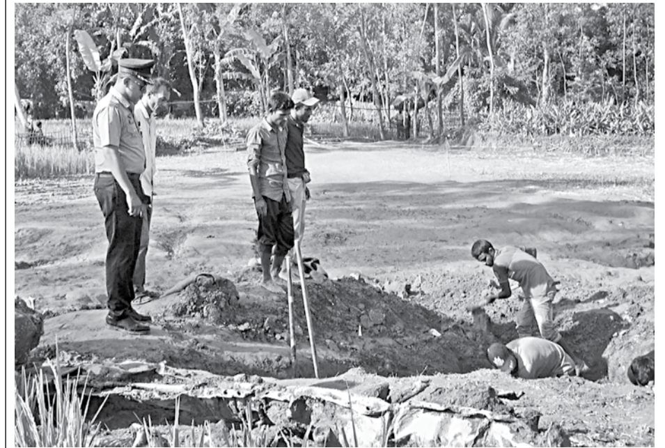
A metal part of the warplane, above, recovered in Lalmonirhat Sadar upazila on Friday. Bangladesh Air Force was digging the farmland to unearth the remains of the warplane.
