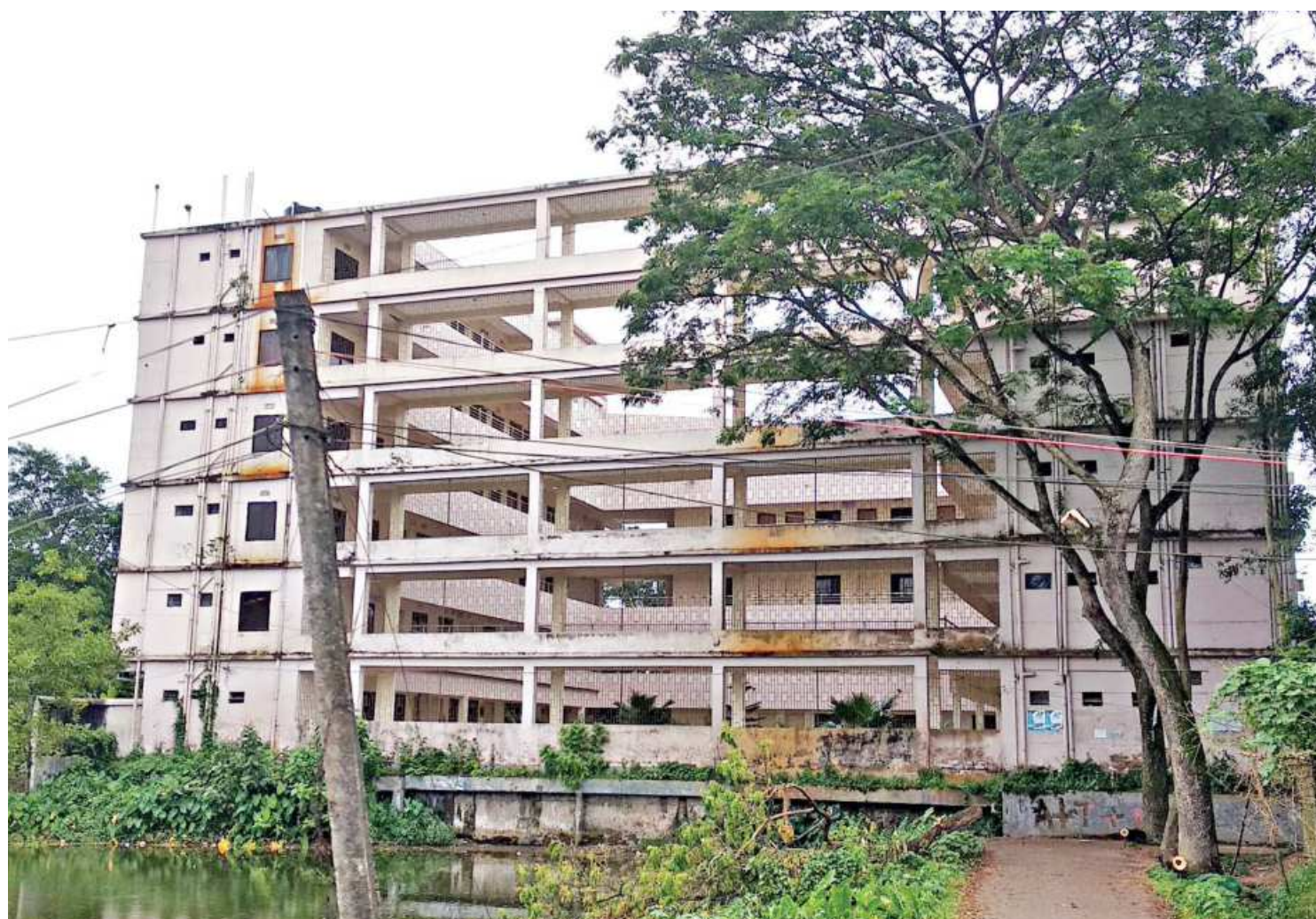
The six-storey Diabetics and General Hospital in Habiganj Sadar's Mashulia area was built on occupied land of the Old Khowai river. It is one of several large buildings and offices set up by the government and influential local bodies on illegally occupied river land.
