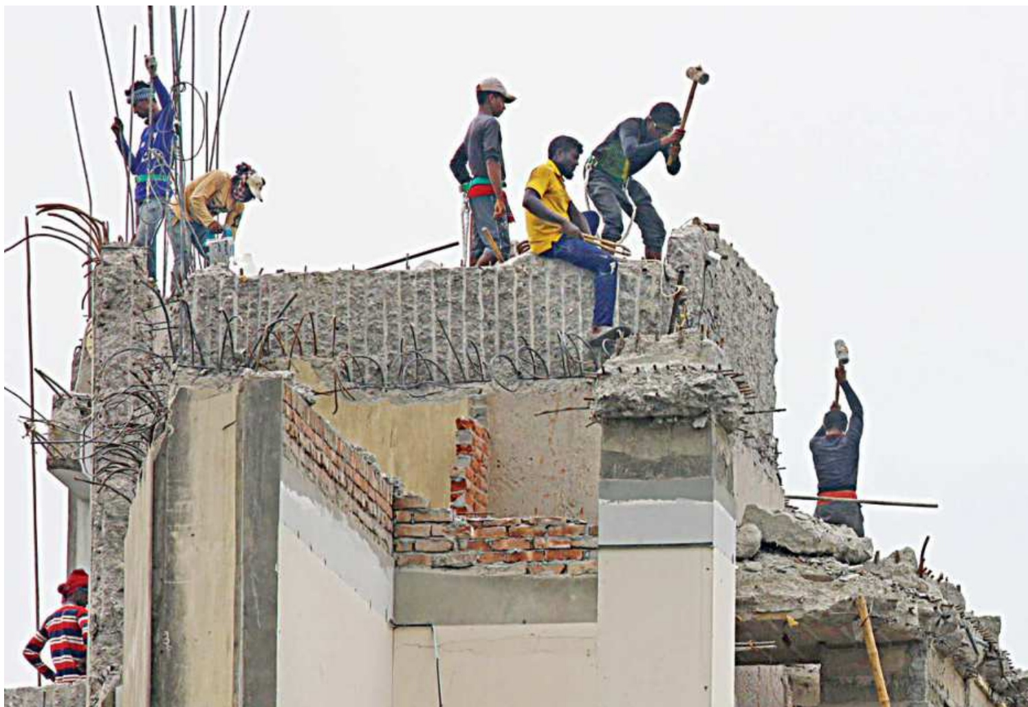
Some of the workers demolishing the illegal BGMEA building have no gear to save them from falling off the high-rise building. Tragedies at construction sites are all too common because of such utter disregard for safety.
