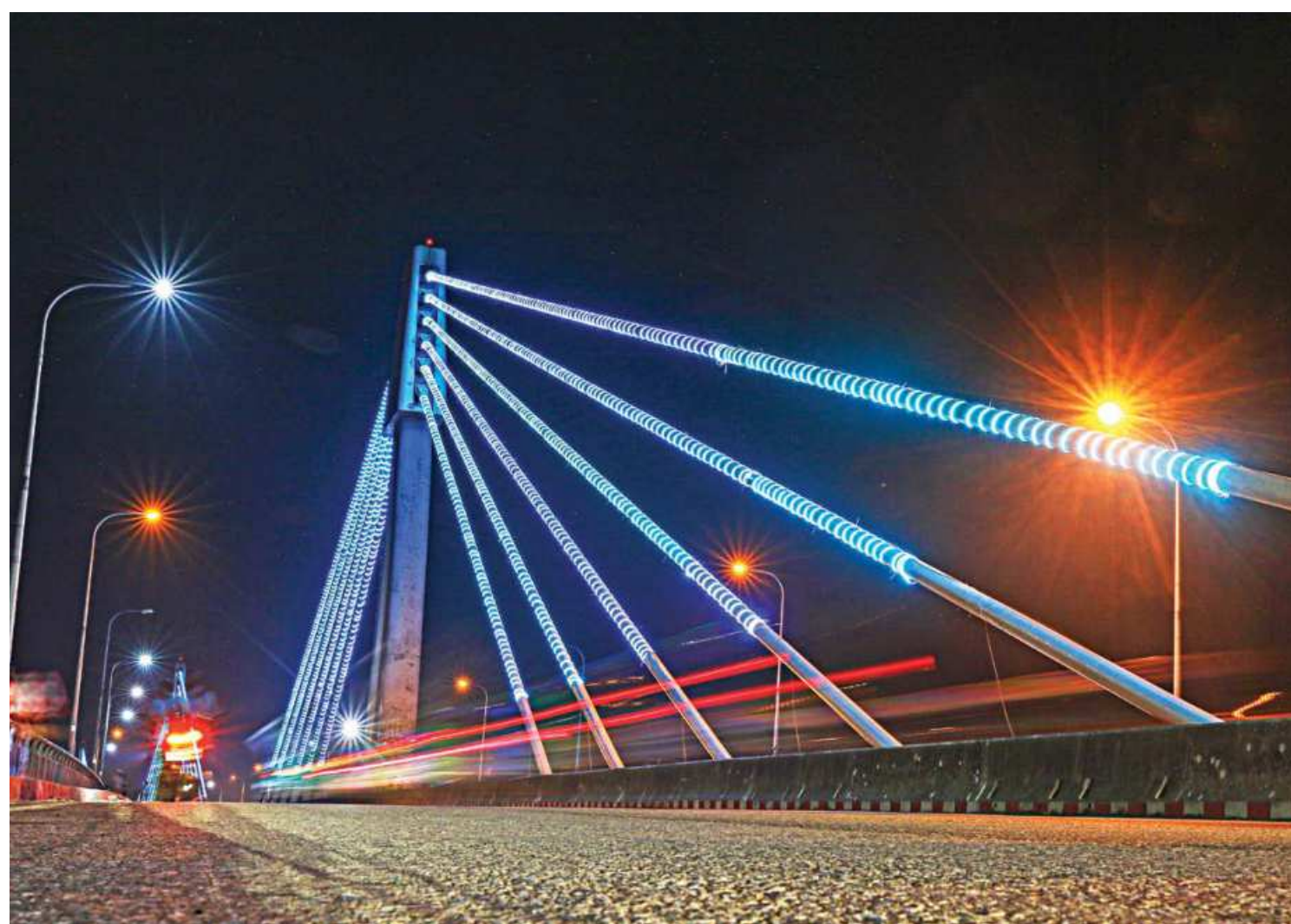
The Shah Amanat Bridge on river Karnaphuli in Chattogram wears a gleaming new look, as the Roads & Highways Department last week completed decorative lighting on the bridge. Officials said the work was undertaken marking Mujib Borsho, and was halted for a few months due to the Covid-19 pandemic. The photo was taken recently.
