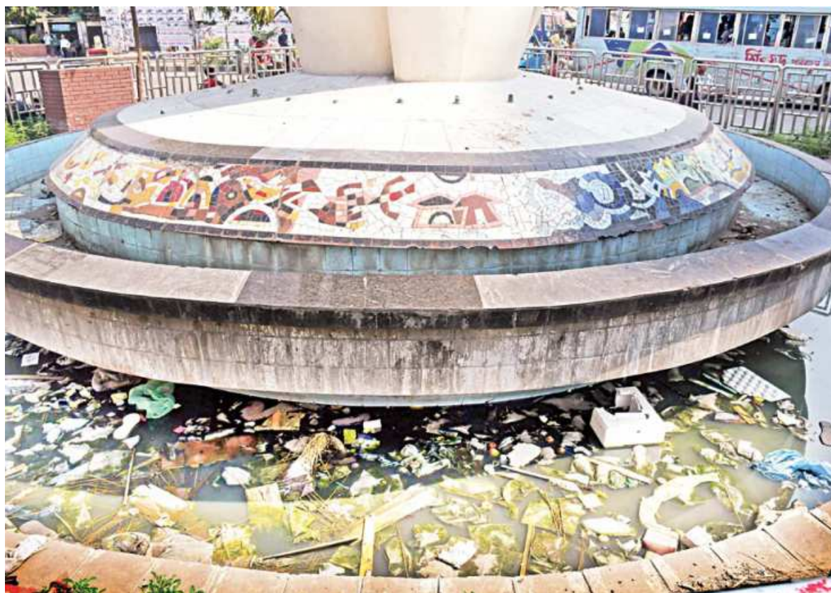
The water in the moat surrounding the Bangabandhu Square Monument in Gulistan is filled up to the brims by trash. Whereas an installation such as this one should make people feel glorious, there's this depressing aura all around the monument. This photo was taken last week.
