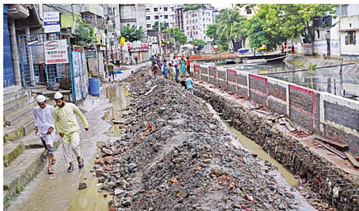
Development work at this two-kilometre road in Mohammadpur -- stretching from Mohammadia Housing all the way to Beribadh -- has been going on for over a month. For more than two weeks, the road has been cordoned off for the works. This is causing immense suffering to the residents of the densely populated area, especially due to the rainfall of the last few days.
