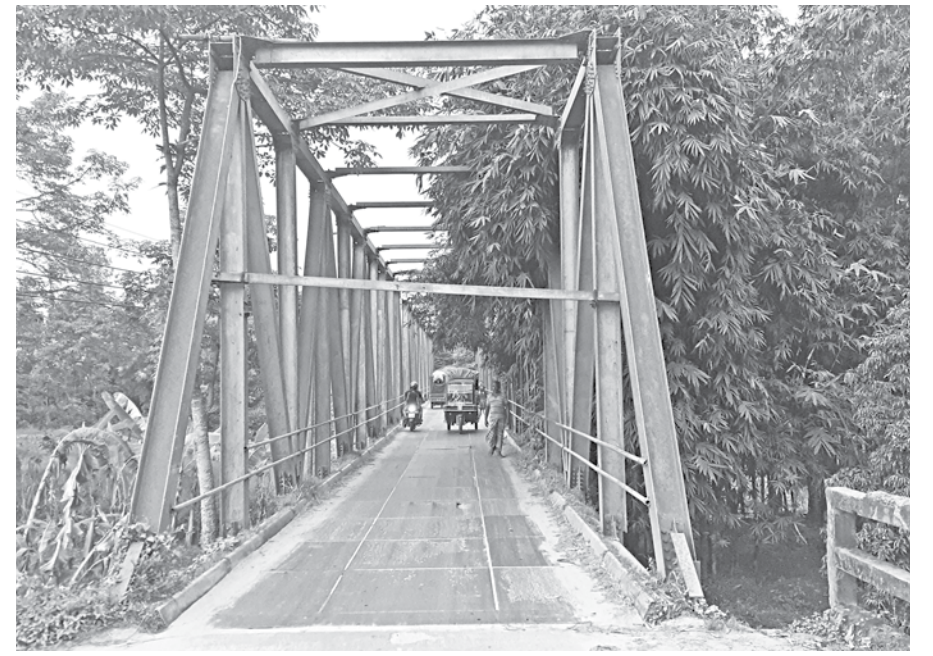
The Bailey bridge in Kulaghat area of Lalmonirhat Sadar upazila.
