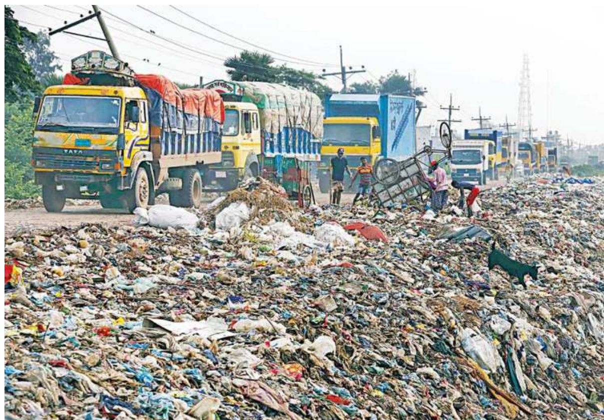
Locals dump waste on both sides of the Asian highway in Jajor area of Gazipur on a regular basis. With time, the dumped waste narrowed down the highway and has not only become a hazard for road users but also for the locals. The photo was taken yesterday.
