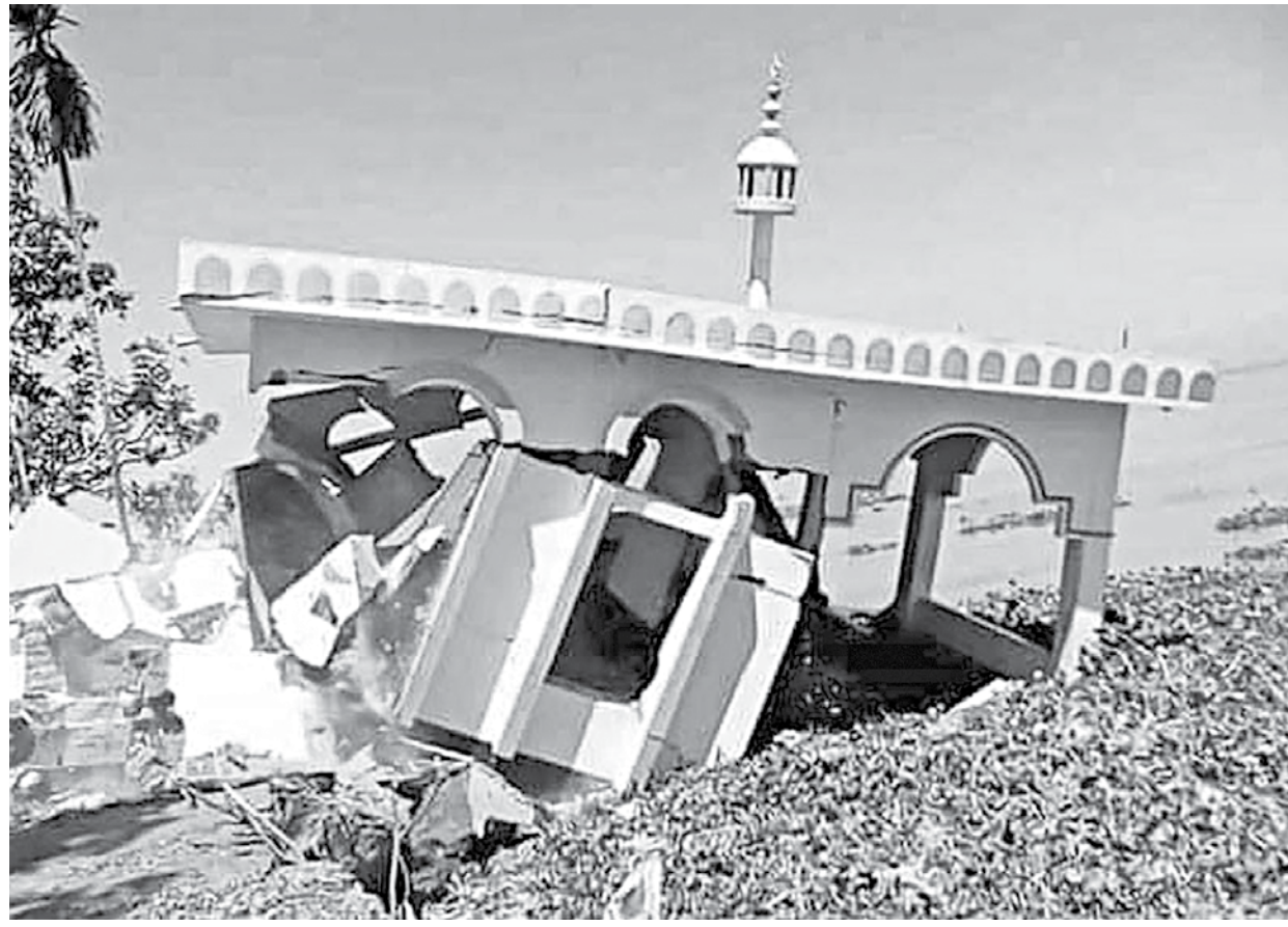
A mosque in Panchthakuri village of Sirajganj Sadar upazila tumbling down as the mighty Jamuna river continues its onslaught on its banks in the area. Along with the mosque, which was the only concrete structure in the village, 10 to 15 houses were also washed away by the river on Saturday.
