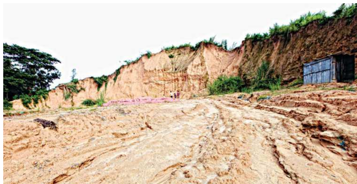
A large portion of this hill in near Sylhet's Pathantula-Madina market has been cut. Locals allege that the hill-cutting work is done by men working for an influential local in the dead of night. This photo was taken recently.
