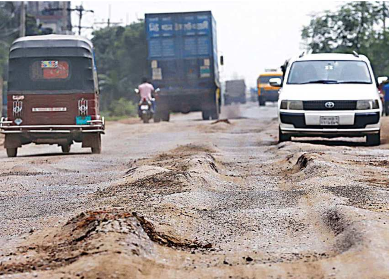
Vehicles ply on Asian Highway in Gazipur's Jajar area that has suffered serious rutting -- grooves created on the surface by overloaded vehicles. The highway is in such a poor shape at different points that it causes frequent tailbacks. The photo was taken recently.
