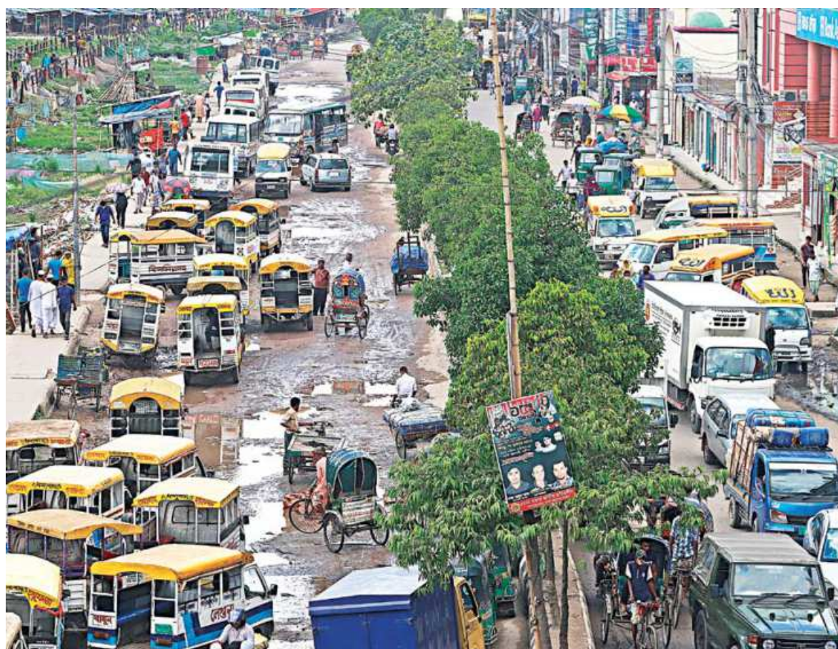
This road in Jurain Railgate area of the capital has become a virtual human hauler stand, and for good reason too. The dilapidated carpeting on the road with puddles all over has left it unfit for vehicular movement. Locals say the situation has been like this for a long time.
