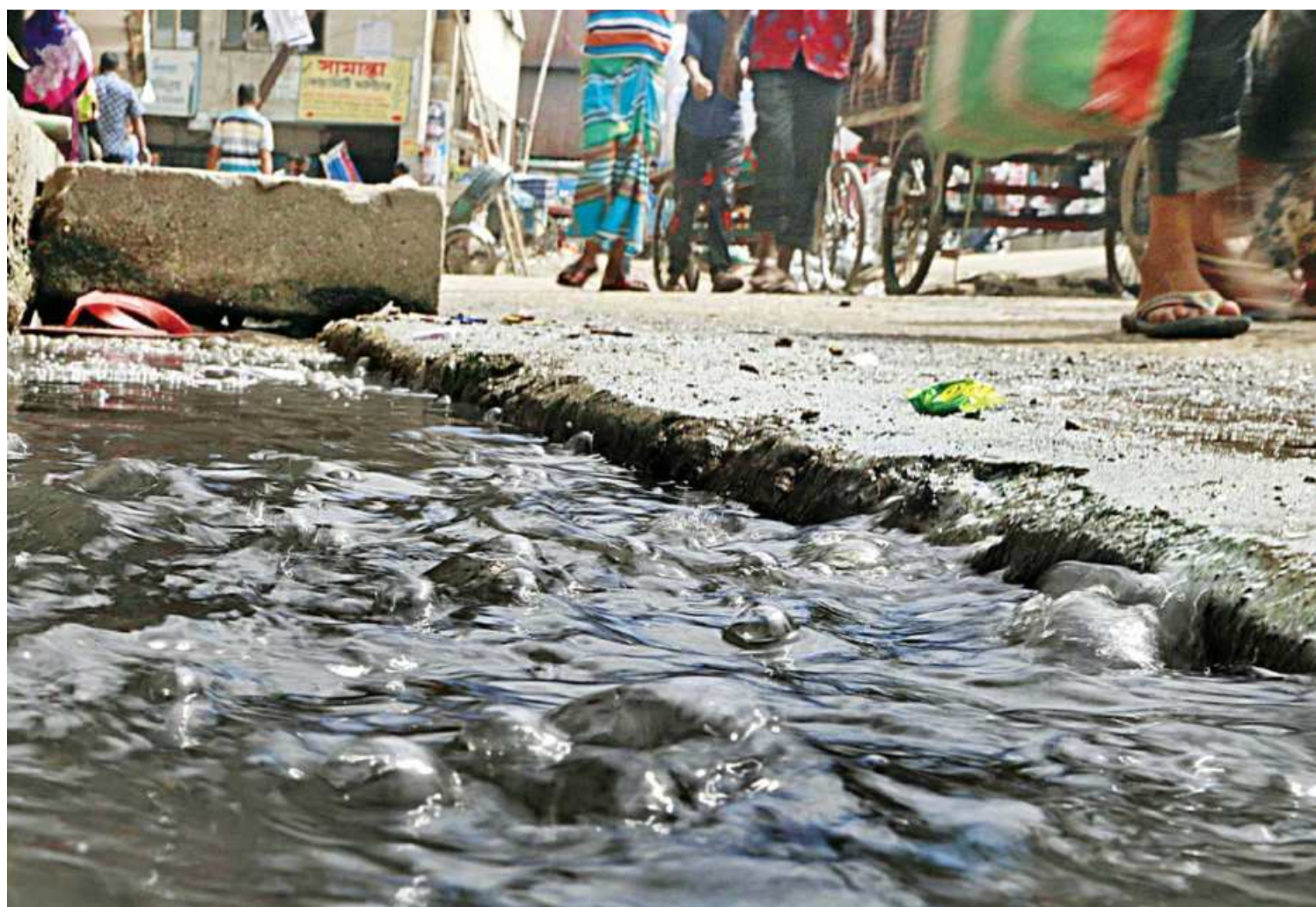
Gas bubbles forming in this roadside drain near Alam Market in the capital's Jurain. A gas line runs parallel to this drain and the leaking gas has created an overpowering odour, but no action is being taken despite complaints from locals. This photo was taken on Saturday.
